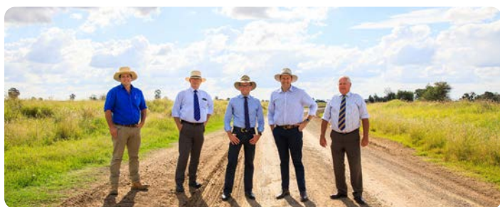
Inspecting the IB Bore Road, which is about to undergo an $11.54 million rebuild and bitumen seal, Gwydir Shire Council Works Engineer Jamie Wilson, left, General Manager Max Eastcott, Northern Tablelands MP Adam Marshall, Regional Roads and Transport Minister Sam Faraway and Mayor John Coulton
